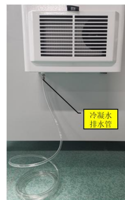
Figure 68: Condensate Drain Pipe of Air Conditioner
