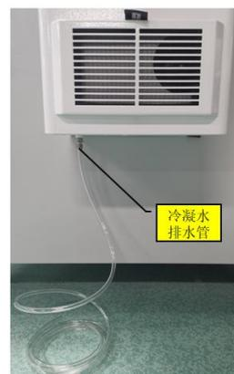
Figure 68: Condensate Drain Pipe of Air Conditioner
