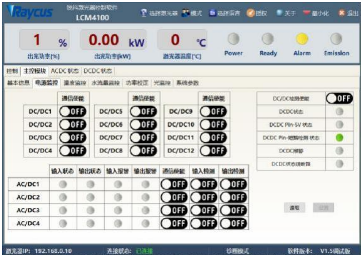
Figure 17 Alarm information interface of main control module
